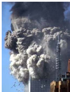
The South Tower’s top tilted 22 degrees, then disappeared straight down into the rubble cloud.
