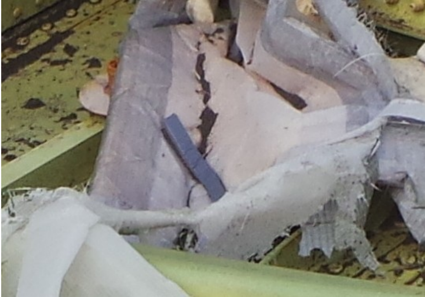
The skin of the lower part of the fuselage, next to the second door on the left Source
